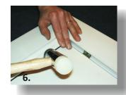
On some systems it may be necessary to notch centre pips and double leg beads around the Securi-Panel to obtain a flat base.
