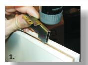
With the Aluminium Skin to the outside, tap Securi-Panel into position 60mm from corner to edge of clip
